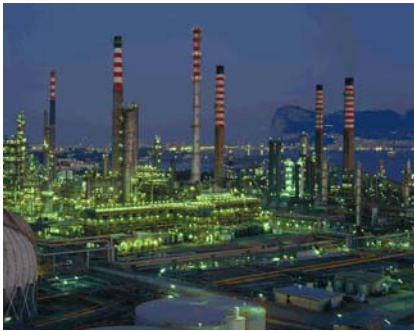
Figure 3 : CEPSA industrial plants in the bay of Algeciras
